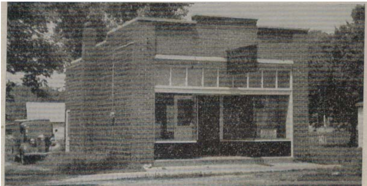
A store building is converted into a honey house by Earl Robinson, Oelwein, IA - 1943
